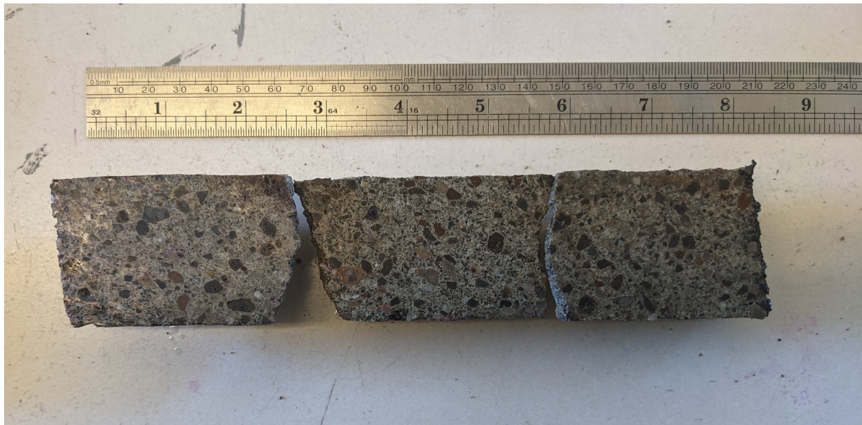
Figure 2. CMU reference core section after application of the phenolphthalein indicator (freshly cut cross section). No color change was observed, which indicates a pH <10 and carbonation of the cementitious paste has occurred throughout the CMU block.
